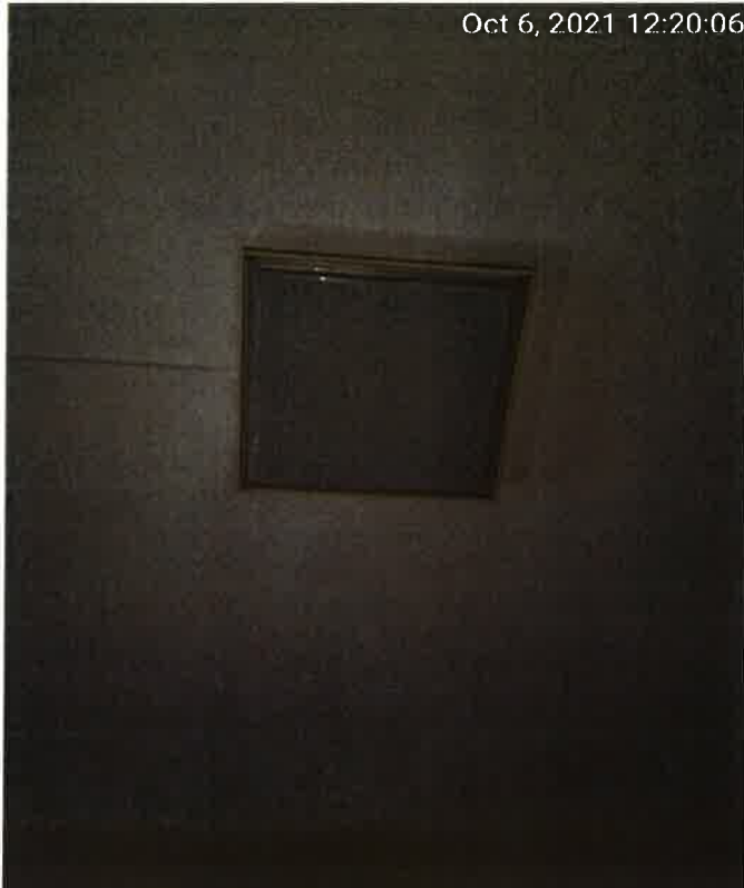
2 ROOF ATTACHED LAMPS
