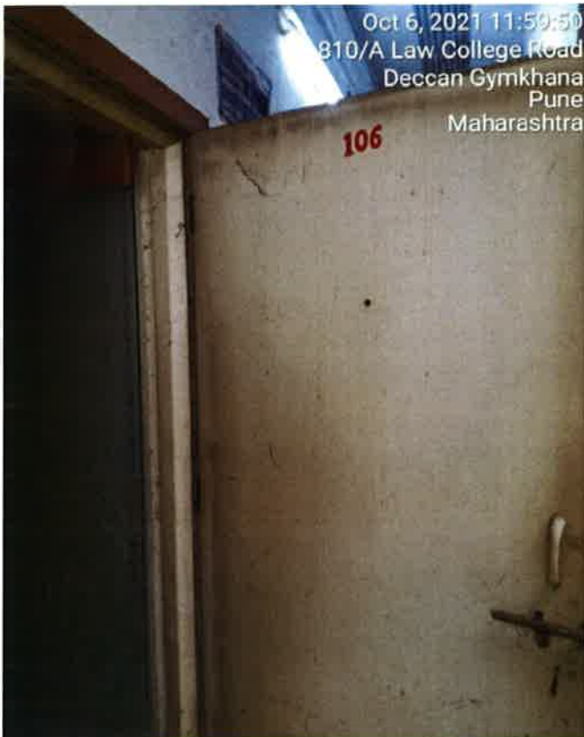
OFFICE ENTRANCE DOOR PHOTO
